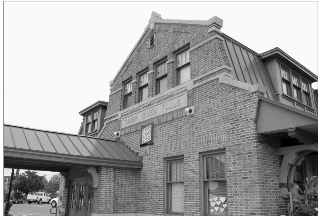
A portion of the Thief River Falls City Hall Back then, it cost $60,000 to build the depot. was used as a depot and completed in 1914.
