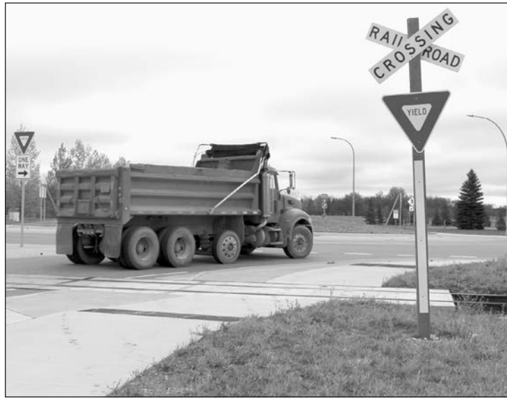
Signals and stop arms will be installed this month at this railroad crossing, which runs through one leg of the Highway 32 roundabout. The project is estimated to cost $245,977.17.
