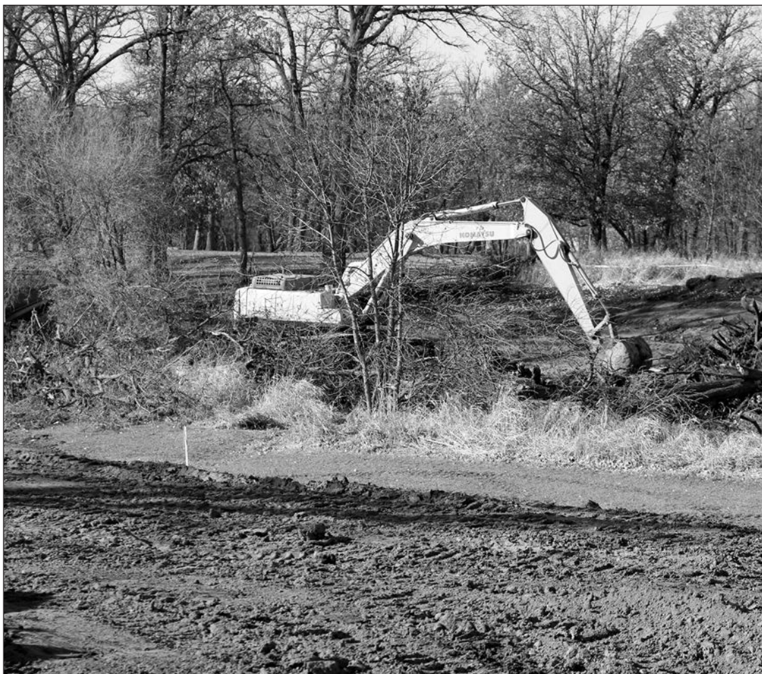
Trees and dirt were removed from an out of bounds area east of the 18th fairway at the Thief River Golf Club. The dirt was loaded into a dump truck and dumped on the 18th fairway to raise the surface above minor flood stage.
