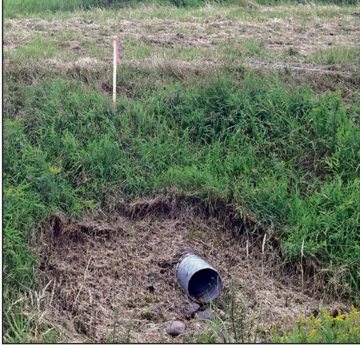
Forty-three side water inlets were installed along 15 acres (1.25 miles) of land near Thief River Falls. The average buffer width was also extended to 46 feet. The project cost nearly $130,000 and included funding from a variety of sources.
