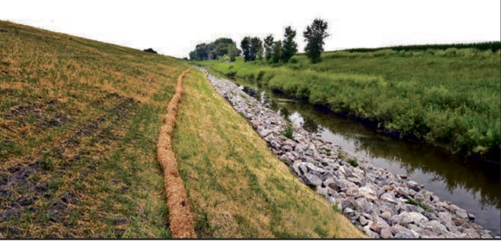
This shows part of Phase II of the County Ditch 96 project. Nearly one-half mile of the south bank was stabilized by the project. It involved several funding sources.
